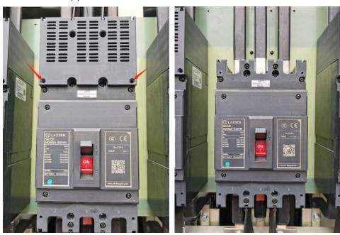
2) Remove the copper bars and cables connected to the upper and lower ends of the molded case circuit breaker.
