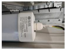
2) Remove the lamp fixing screws (M6 external hexagonal bolts) and remove the lamp.
