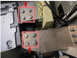
2) Remove the signal cable and grounding cable of the air circuit breaker and mark them.
