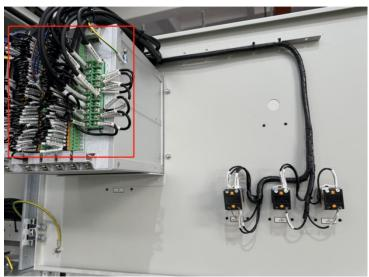
3) Remove the screws that fix the device, and remove the device (M6 external hexagonal bolts).
