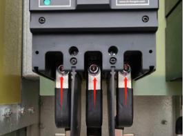
3) Remove the fixing bolts of the molded case circuit breaker and remove the molded case circuit breaker.
