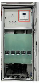
2) Open the cabinet where the device is located, remove the cables on the back of the device, and mark the recording location; You can also remove the entire plug-in terminals and install them in the corresponding position of new devices.
