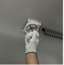
2) Insert the new smoke sensor into the base and rotate it clockwise to the locking position.
